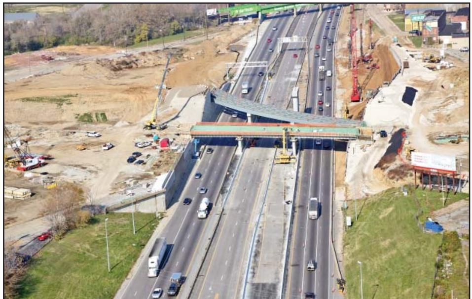
**Girders line the new ramps and bridges over I-70 just north of Cass Avenue leading to the new Mississippi River Bridge. Drivers should expect summertime lane and interstate closures to put the driving surfaces on these bridges.**
