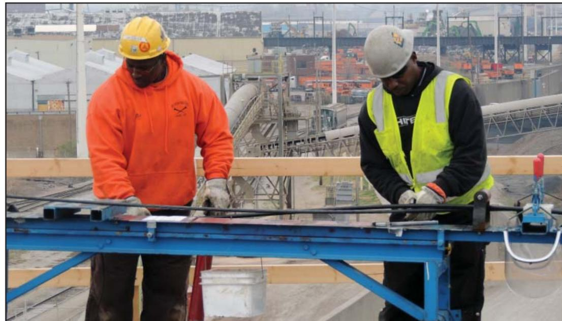
Ironworkers prepare the cable before it is installed inside a conduit.
