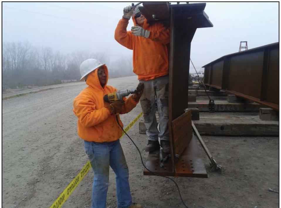
**Crews prepare girders before building a section of the bridge support structure.**
