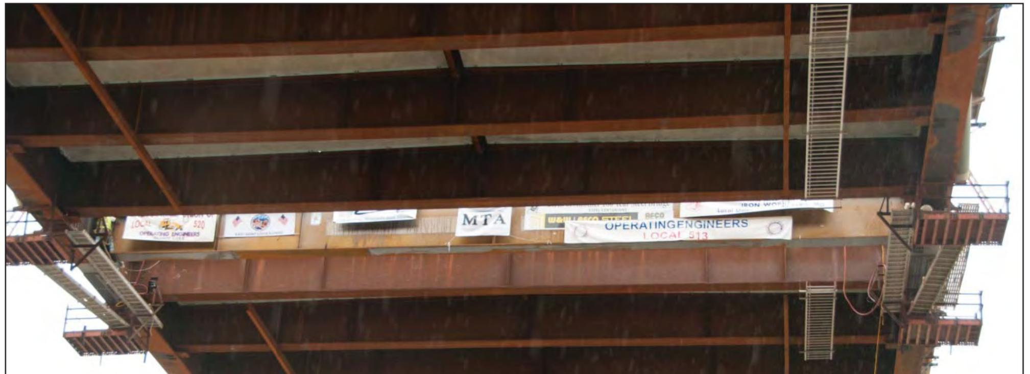
The final floor beam is set into place on the new bridge. The 80-foot long beam weighs roughly 30,000 pounds.
