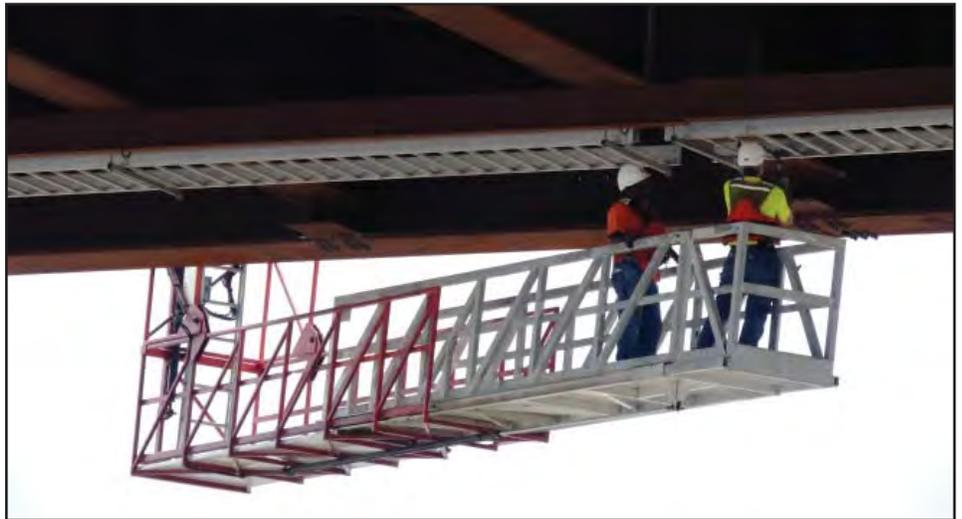
**Electricians from BRK Electrical Contractors install the cable tray system on the underside of the new Mississippi River Bridge.**
