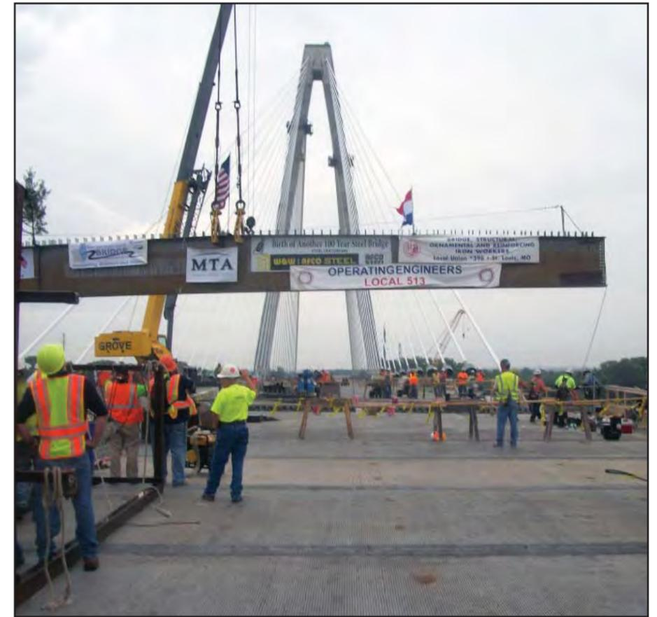
The final floor beam swings into position
