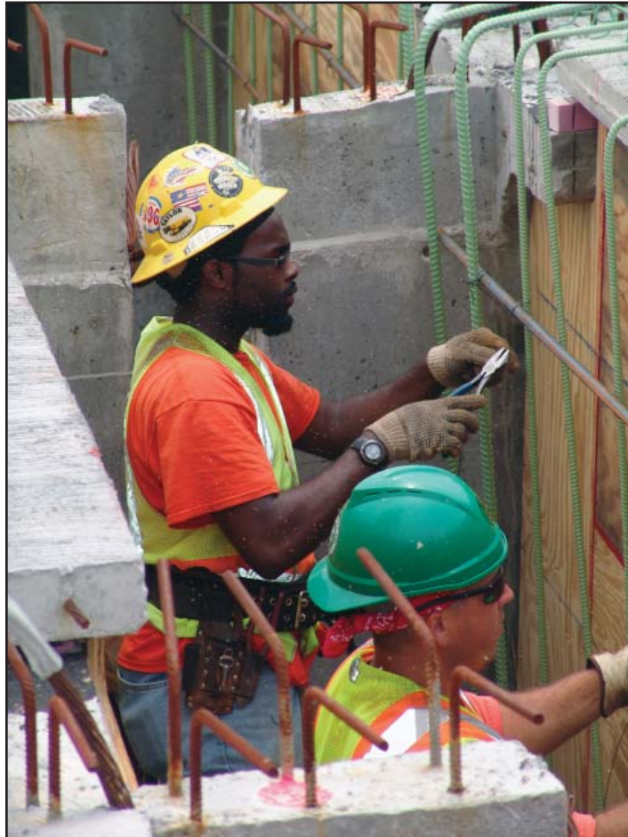
Ironworkers place reinforcing steel on the Missouri Approach.
