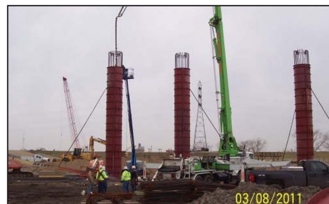
Illinois crews pour concrete for the Illinois Approach foundation work.
