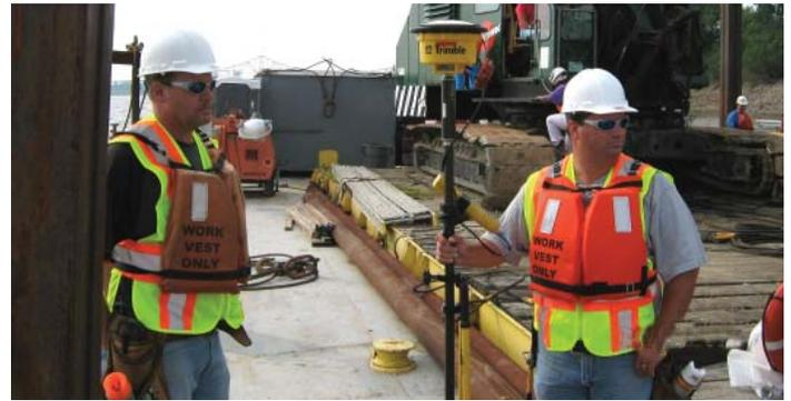
**Jeff Geisen, left, and Jeff Hull of Engineering Design Source, Inc. stake borings for the Mississippi River Bridge foundation piers, while on a barge in the Mississippi River.**
