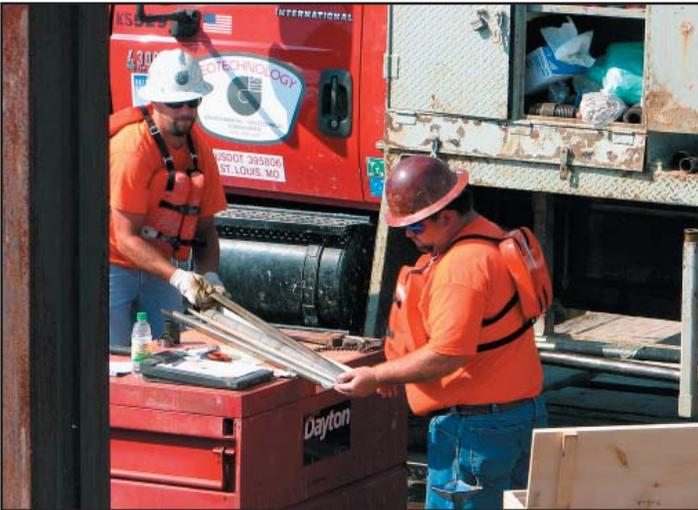
Crews remove a sample of limestone from the drill to package for analysis.
