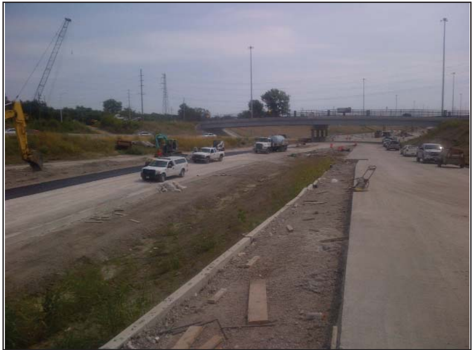
Construction crews rebuild the ramp at eastbound I-64 in Illinois.
