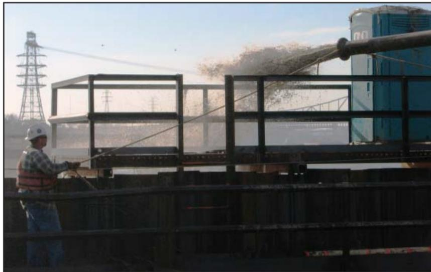
Crews use a pump to remove water from the cofferdam while pouring 3,000 yards of concrete.
