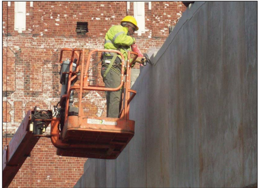
Harry Ballard, new journeyman, prepares a foundation cap for girders.
