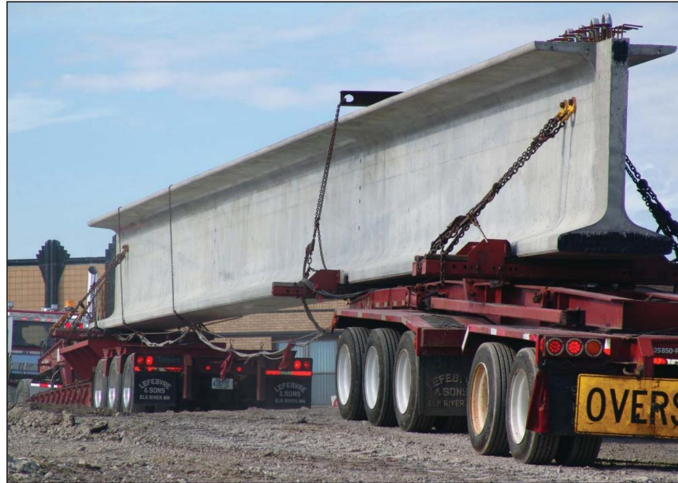
A driver backs one of the massive girders into position to get lifted into place.
