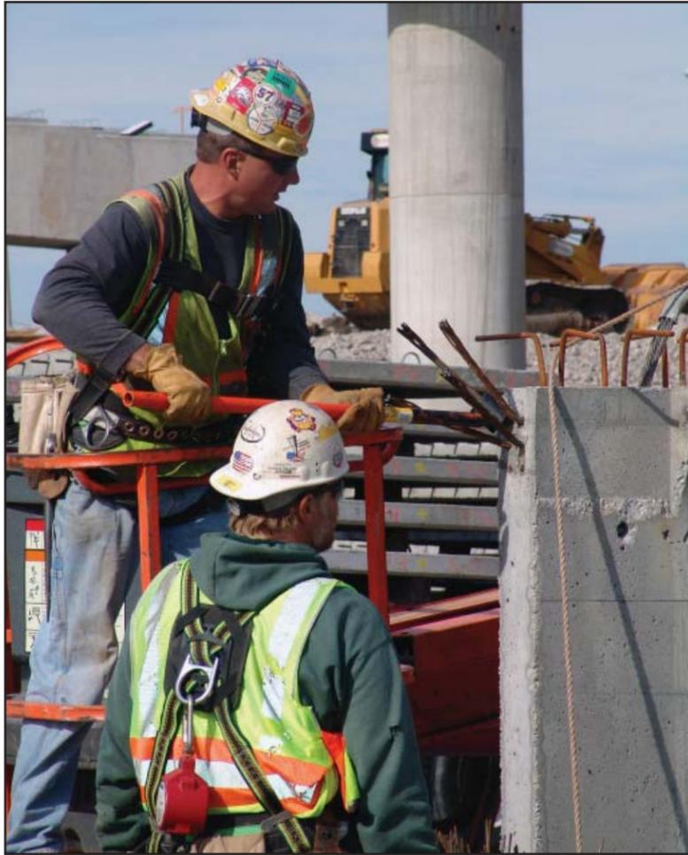
Workers straighten reinforcing steel on a girder before placing it on the Missouri approach.
