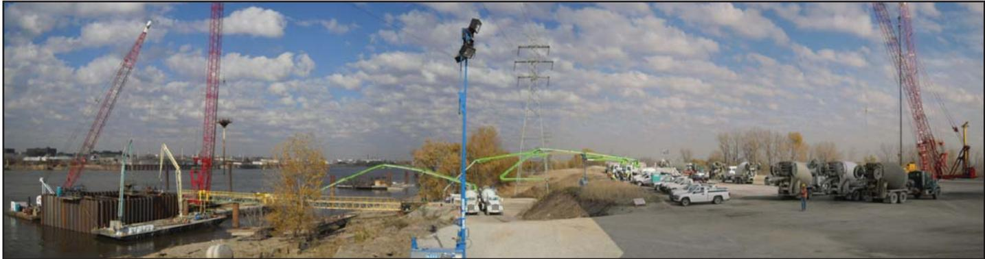
Concrete trucks line up to pour nearly 3,000 cubic yards of concrete for the seal course, part of the foundation for the river bridge project. The seal course gives crews a flat, solid building surface on the river bottom.
