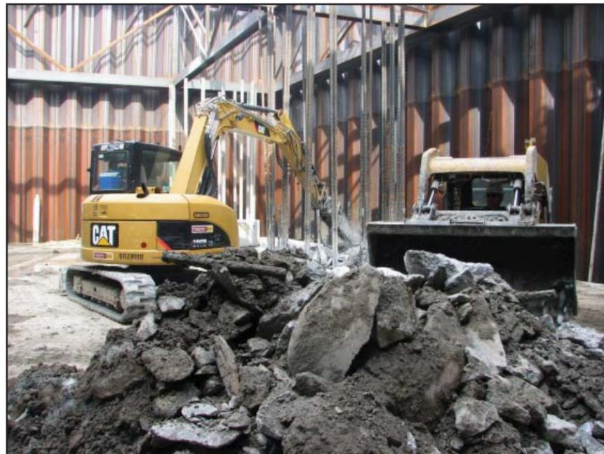
Operators break up and remove the concrete from the floor of the Mississippi River inside the Illinois cofferdam.
