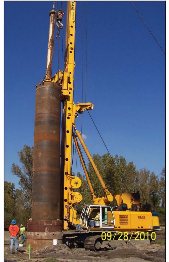
Equipment operators drive a casing into the ground for the Illinois approach.
