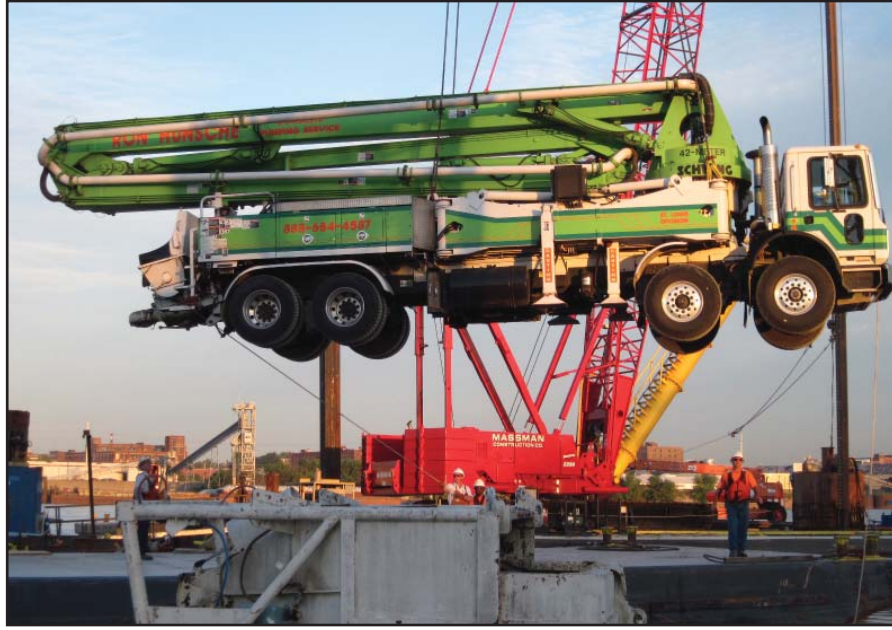
The contractor uses a crane to move a concrete pumping truck onto a barge to pour concrete for a portion of the main span foundation.
