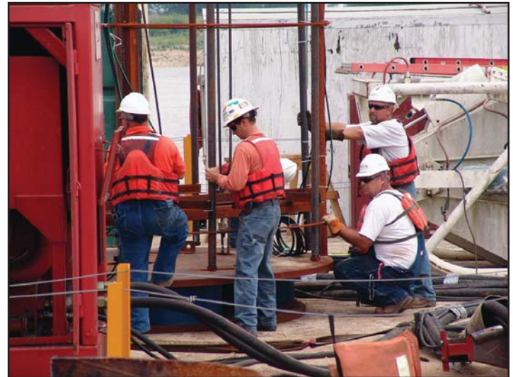
Welders attach the test cells to the framework.
